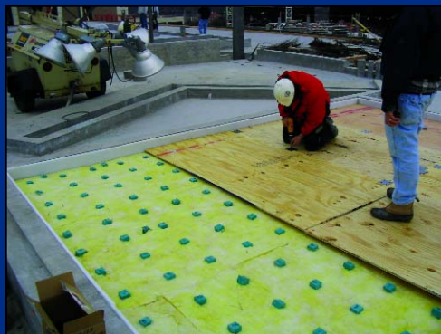
3) Secure junction plates on plywood pouring form
