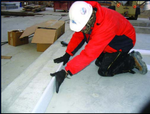
1) Place Perimeter Board (Model PIB)
