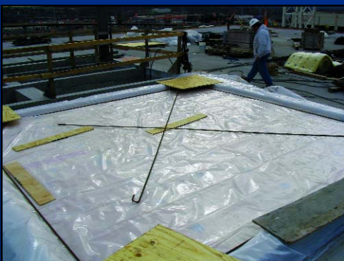
4) Cover with poly layer. Ready to install reinforcement and pour concrete.
