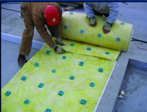
2) Roll-out Model RIM and cut as needed
